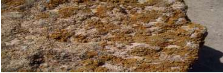
Fig. (15) biodeterioration of limestone
