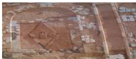
Fig. (12 ) Spallation of marble decoration slabs
