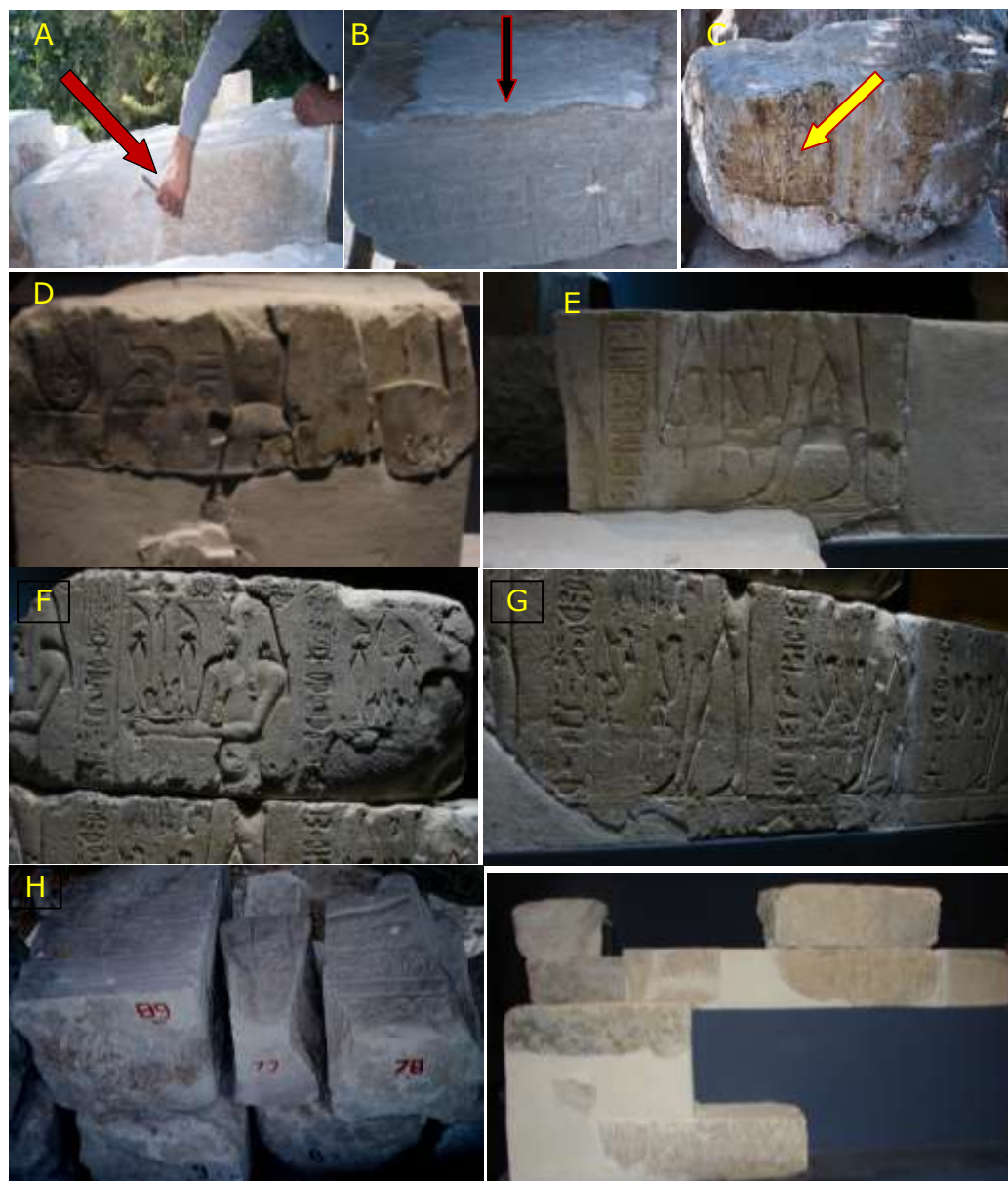
Figure. 23 restorations steps of stone blocks (a) mechanical cleaning (b) absorbent poultices (c) the stone block after poultice. (D,E) Completion of missing parts (E,G) Re-jointing the stone blocks, (H) the blocks after restoration in Excavation field (I)the exhibition of stone blocks at Suez museum.
